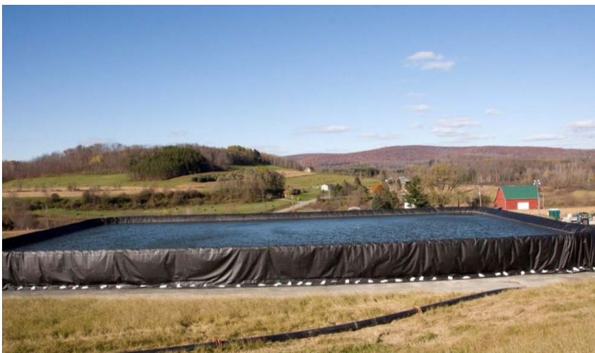
A temporary freshwater impoundment to be used for fracking, or hydraulic fracturing.
